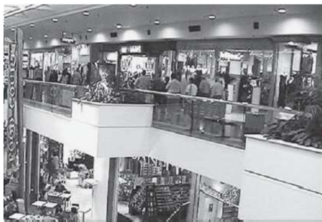
Photo 1: First level shopping centre balustrade
